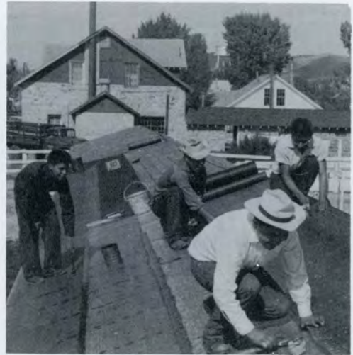
Farm Boys putting a new roof on calve pens
