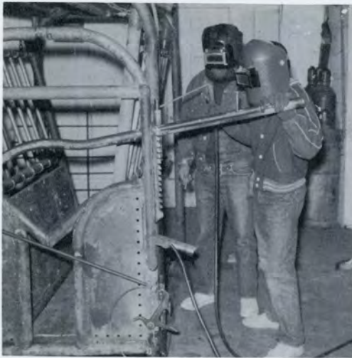
Farm Welders making a branding chute
