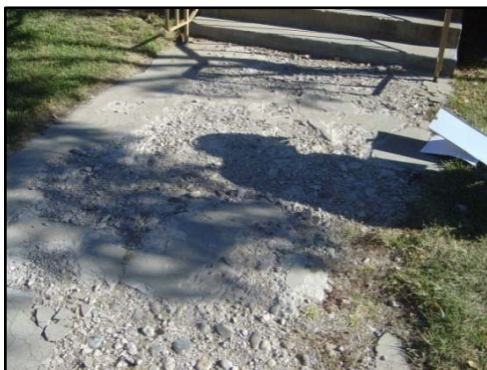
▲ Sidewalk deterioration
